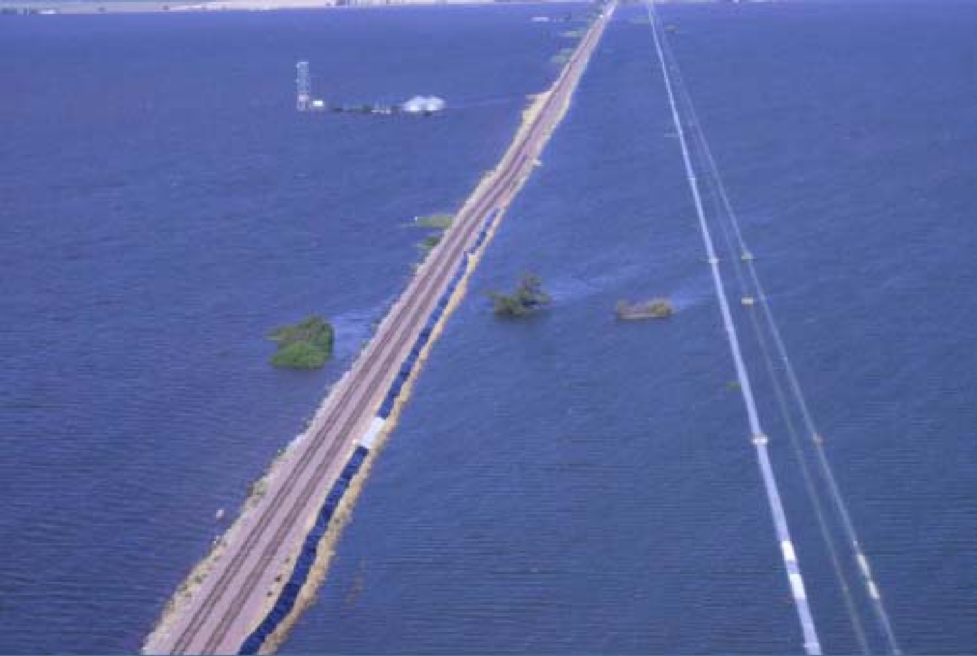
Mokelumne Aqueduct parallels railroad
